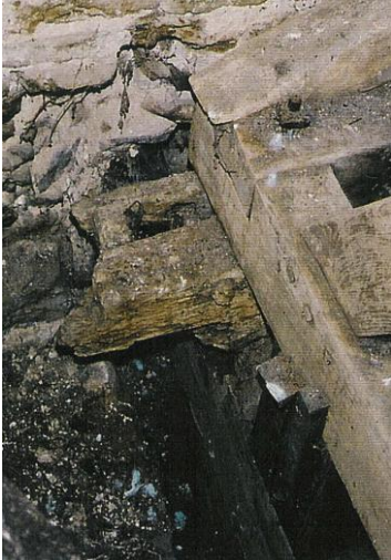
The 1789 frame sat on sills of the 16 th /17 th Century five-bell frame, supported by older primary timbers.
