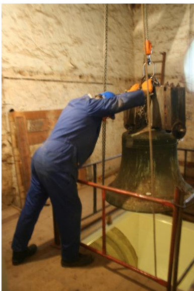
Whites bell hanger lowering through the new trapdoor
