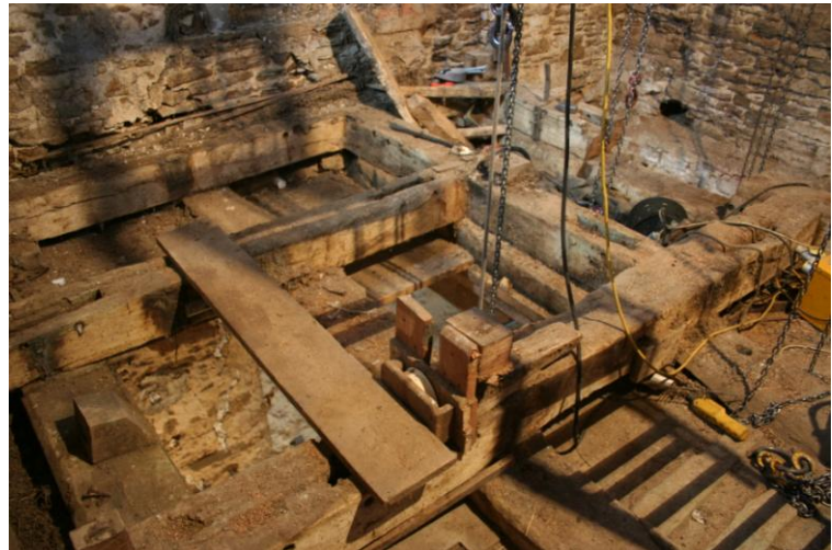
The 1789 frame sat on sills of the 16 th /17 th Century five-bell frame, supported by older primary timbers.
