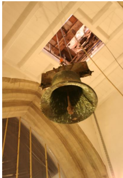
Whites bell hanger lowering through the new trapdoor
